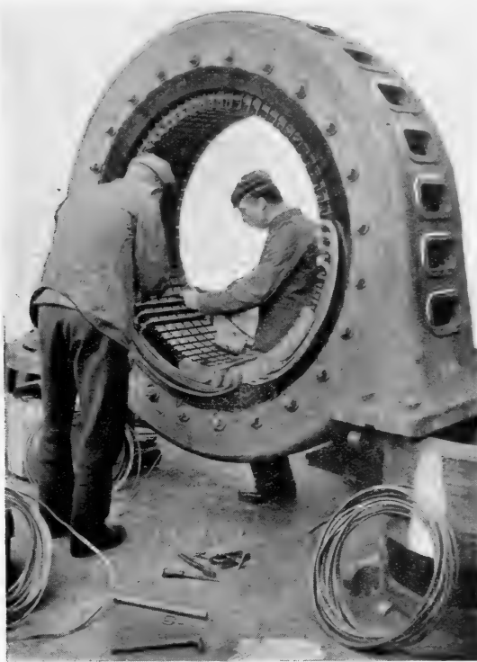
FIG. 390.—Winding Armature with Strip on Edge (Mavor & Coulson).
